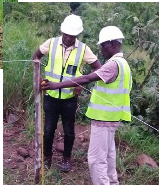
The local foreman and boNGO Director Justin confirming the foundation measurements.
